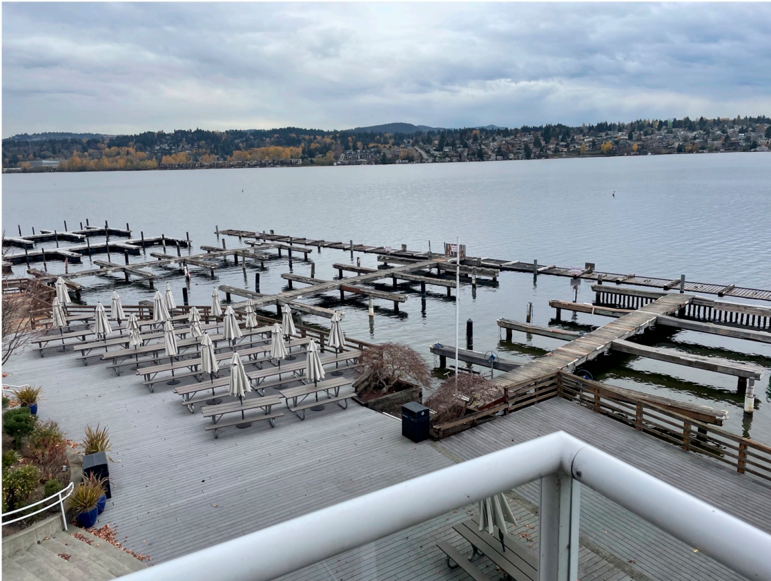
Photo 1 - Existing marina looking waterward.
