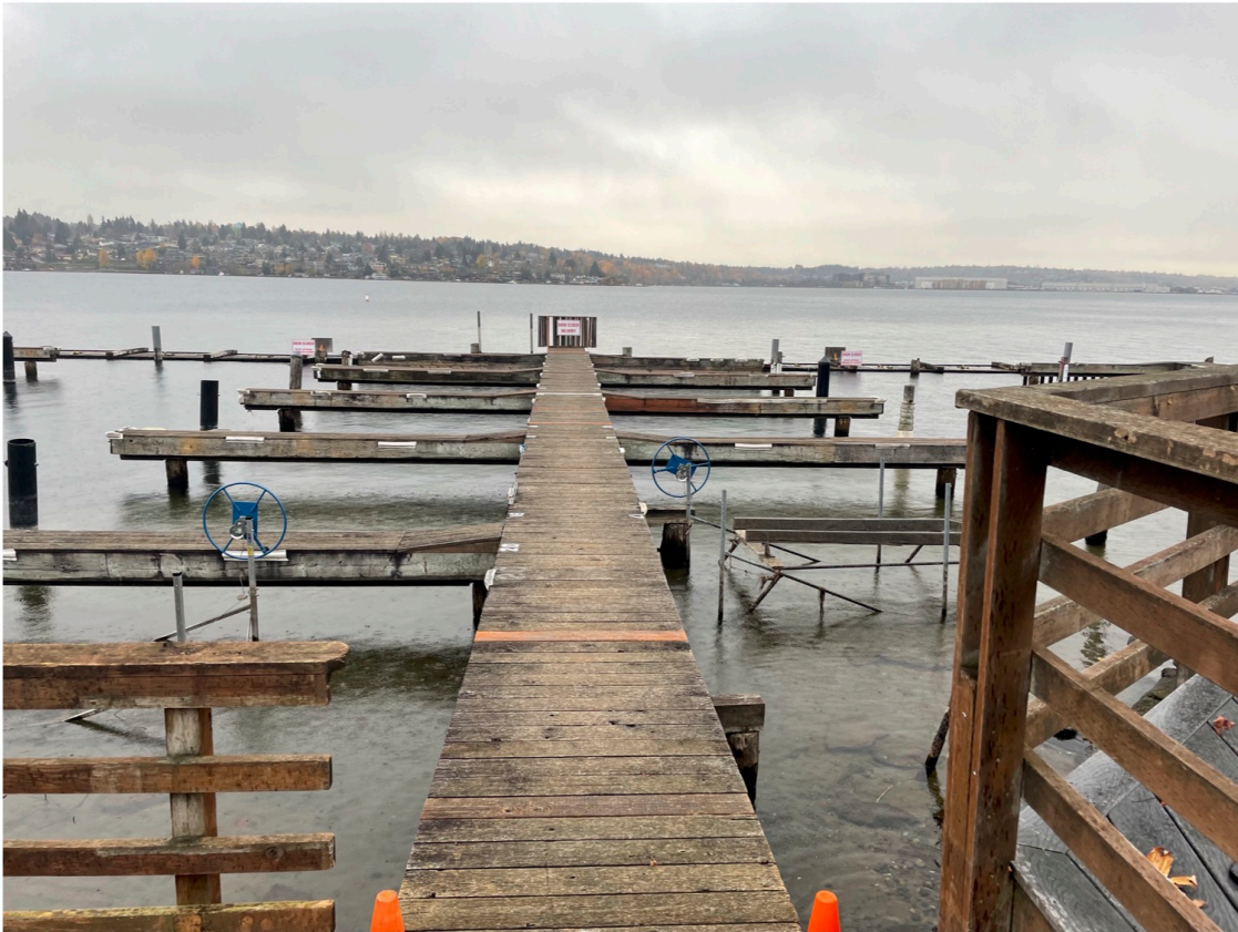
Photo 5 - C-dock looking waterward.
