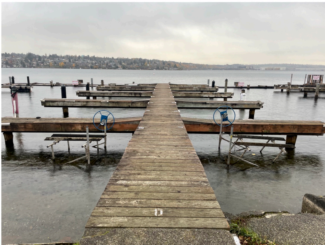
Photo 4 - B-dock looking waterward.
