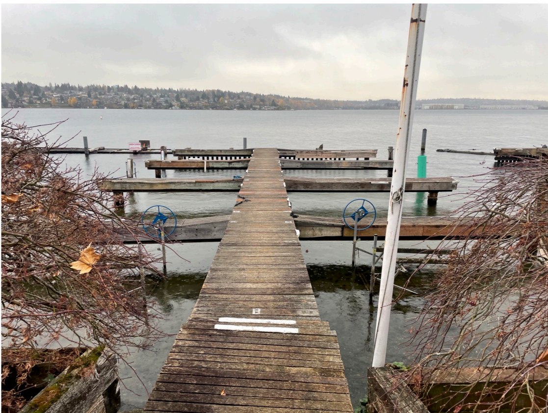
Photo 6 - D-dock looking waterward.
