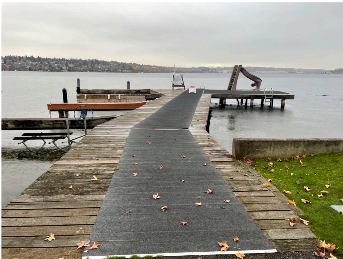
Photo 3 - Existing swim dock looking waterward.
